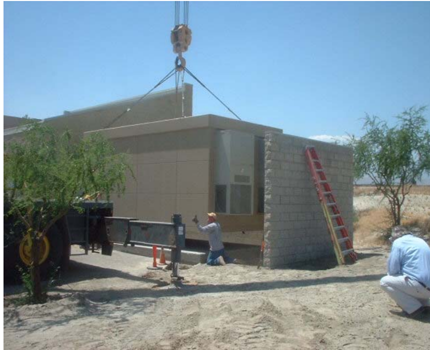
Installation of CalREN Palm Desert Hub Site on CSUSB-PDC Campus
